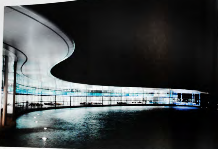
Ahead of the curve The winding glass elevation and cantilevered shading soffits of the Foster + Partners-designed Technology Centre at McLaren's kidney-shaped corporate headquarters in Woking. After its completion in 2004 the building was shortlisted for the prestigious Royal Institute of British Architects Stirling Prize
